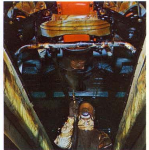
Rust-proofing is also carried out in the body member cavities
